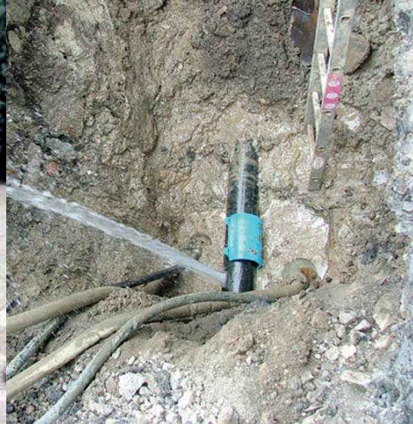
Leakage detection of underground pipelines
