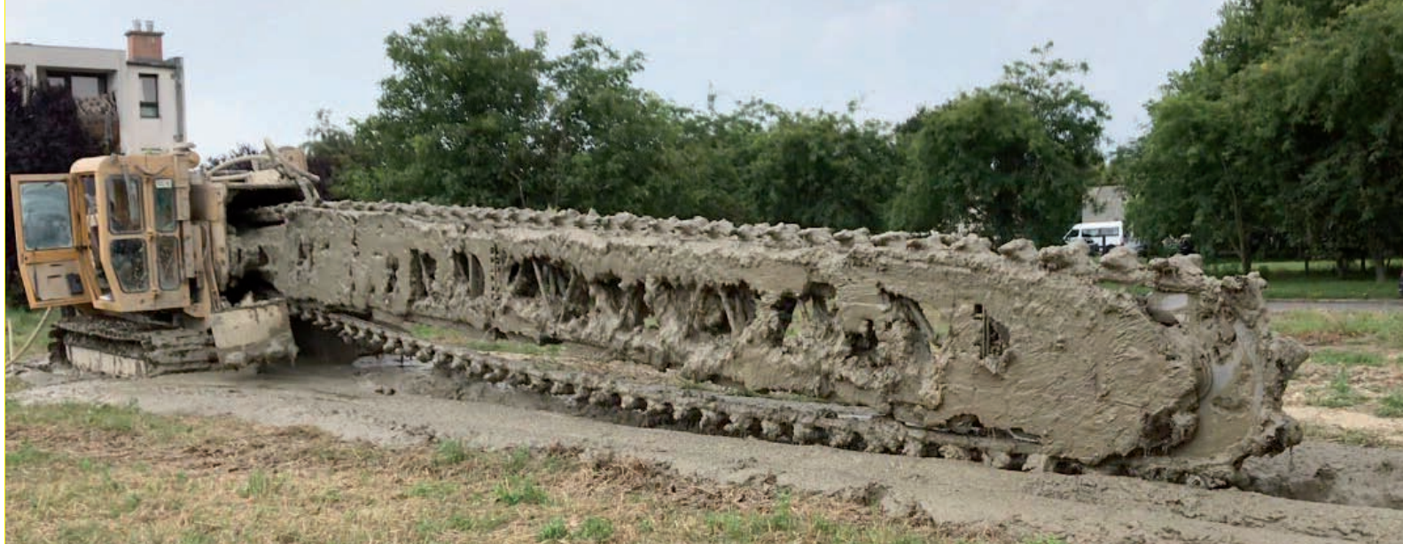
Heavy machinery for waterworks and for groundworks
