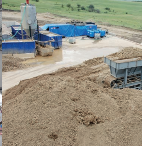
Remediation site with soil cleaning system
