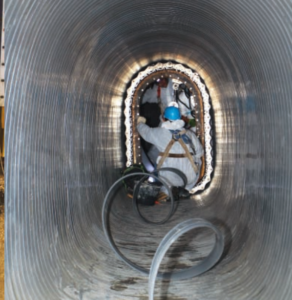
Renovation With SPR Spirally Wound Technology
