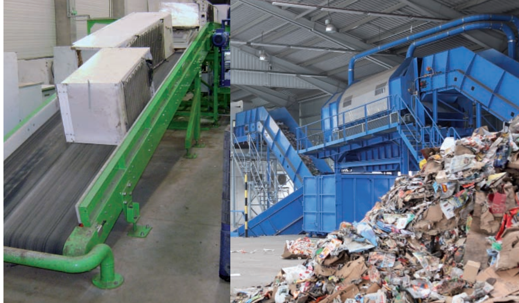
Selective waste processing plant
