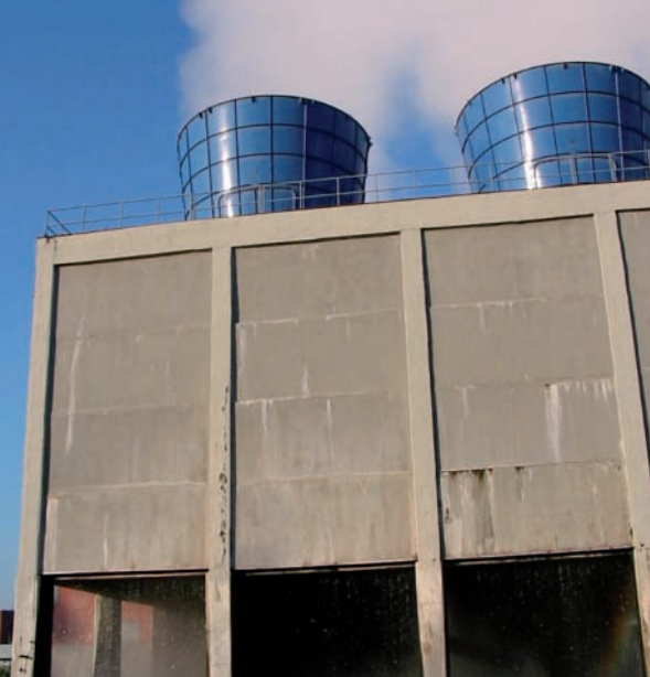
Reconstruction of a cooling tower in a power plant
