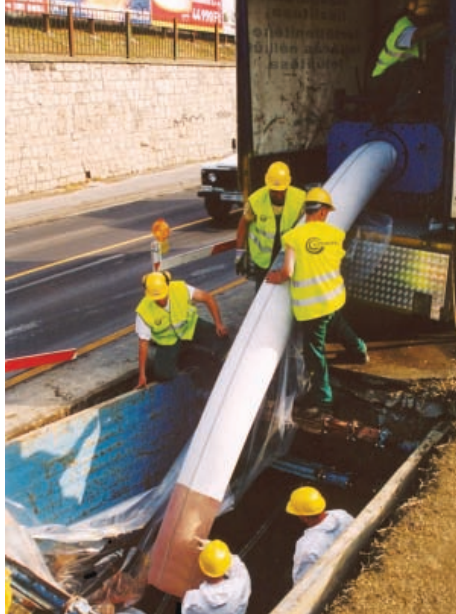
Relining With Process-Phoenix (CIPP) Technology
