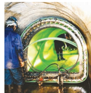
Renovation With SPR – Spirally Wound Technology
